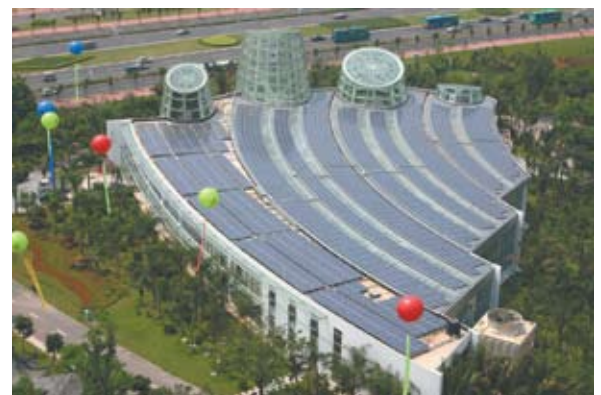
Large-sized system using multiple inverters.
